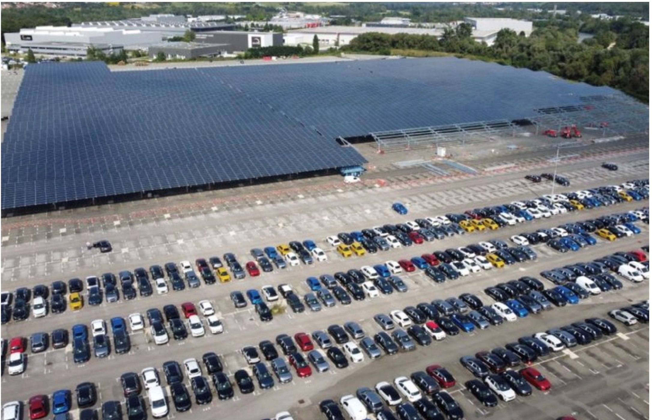
The Peugeot plant in Sochaux has France's biggest solar-canopied car park
